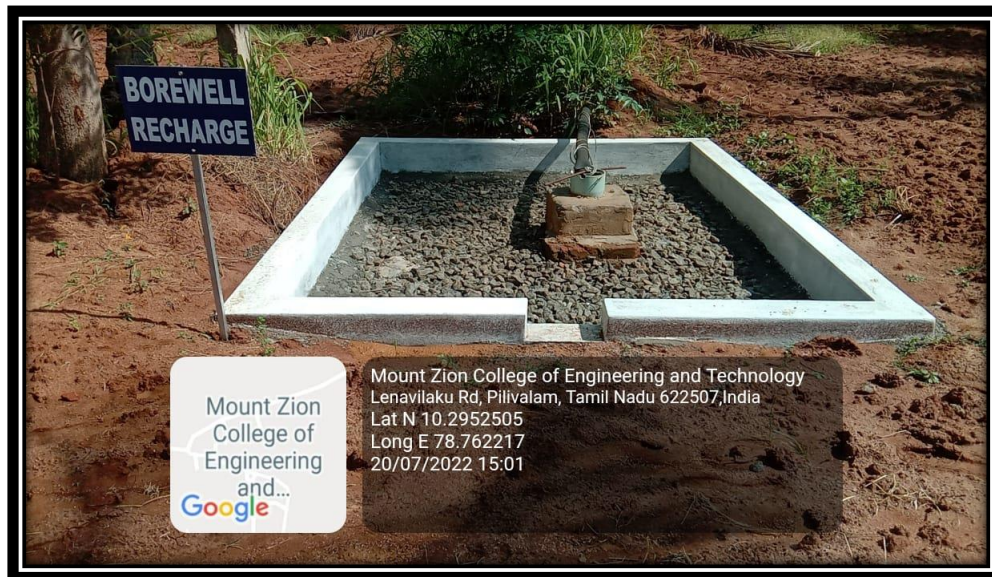
Borewell recharge arrangement near the ground
