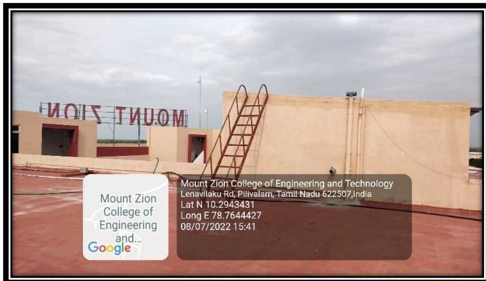
Construction of tank for water supply
