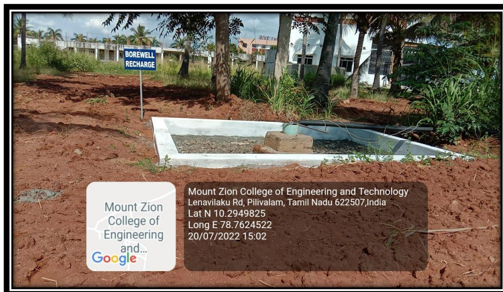
Borewell recharge arrangement near the ground
