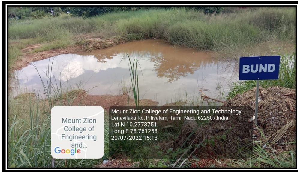
Construction of bunds
